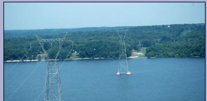
The standard marker balls are virtually invisible until viewed from a location too close to safely respond. Amazingly, this FAA approved marker ball system was put in place without the opinion of pilots. They are a legacy from shipping traffic warning systems, and have been outmoded for years.
